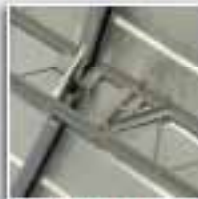
OPEN WEB-JOIST TRUSS SYSTEM PROVIDES ROOF SUPPORT
